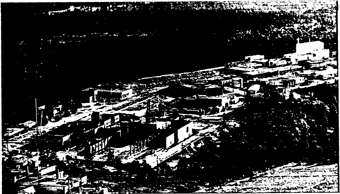
Construction of Antares, LASL's 100 kJ laser system is well under way. Completion of this 62.5-million-dollar facility is scheduled for early 1984.
